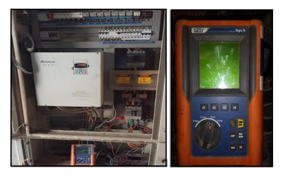
Figure (6.4): Energy analyzer device and collecting data process
