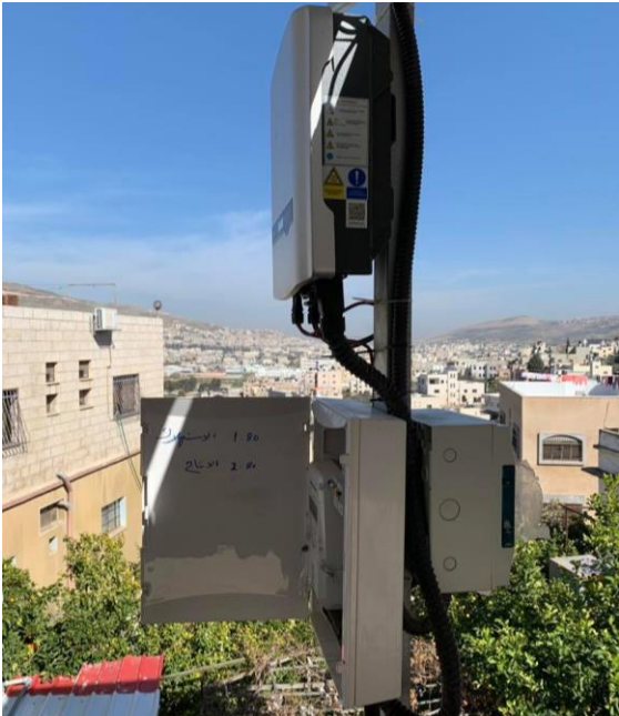
Figure 10:Installing the DB problem
